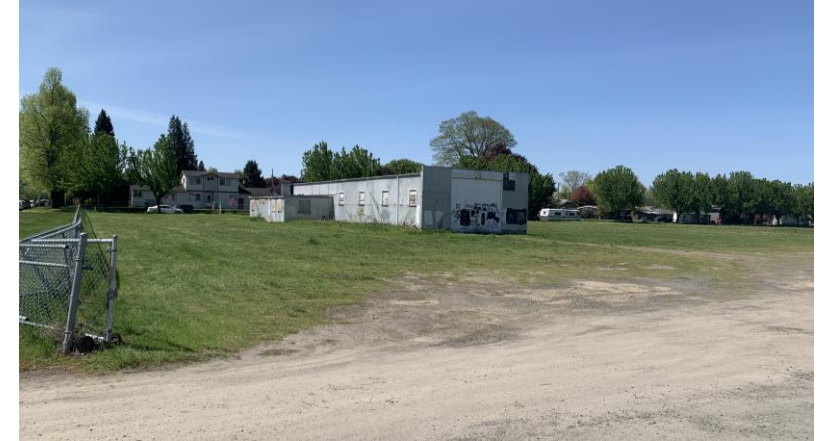
Dilapidated building on the west side of 7 th Avenue
